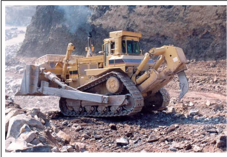
Figure 5: Tracked bulldozer in use on loose ground
