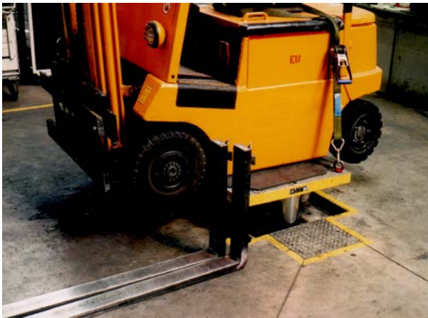
Fig. 35 Lifting forks removed for working on the hydraulic system of a fork-lift truck
