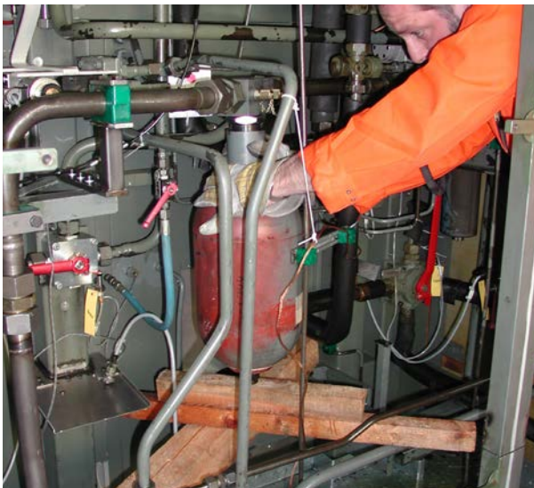
Fig. 1 Maintenance technician during maintenance work
