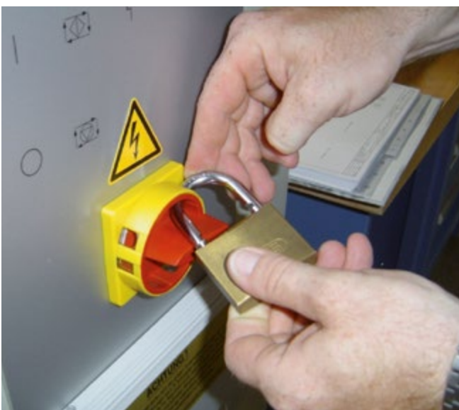
Fig. 58 Electrical energy isolating device [H]
