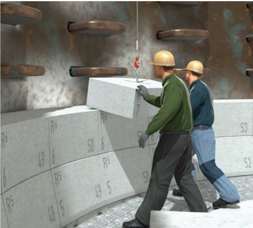
Abb. 77 Transportanker
