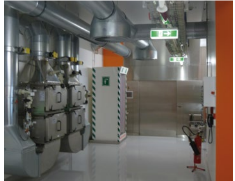
Fig. 4 Building for S3 experiments
