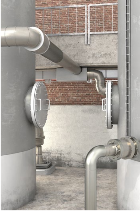
Fig. 12 Manhole (unfavourable position, conditions unfavourable to rescue)
