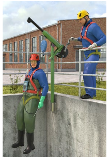
Fig. 25 Access technique involving full body harness and rescue winch
