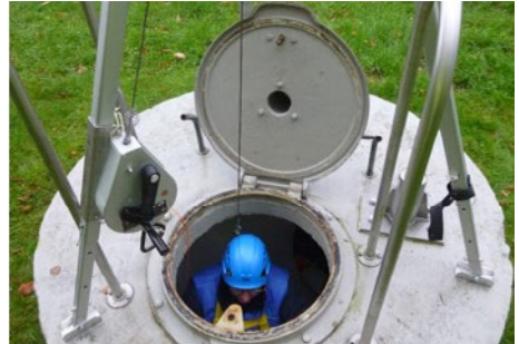
Fig. 23 Retractable type fall arrester with rescue lifting device
