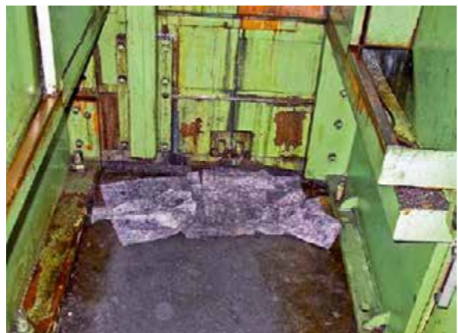
Figure 4 Increased fire load due to cleaning cloths soaked in oil
