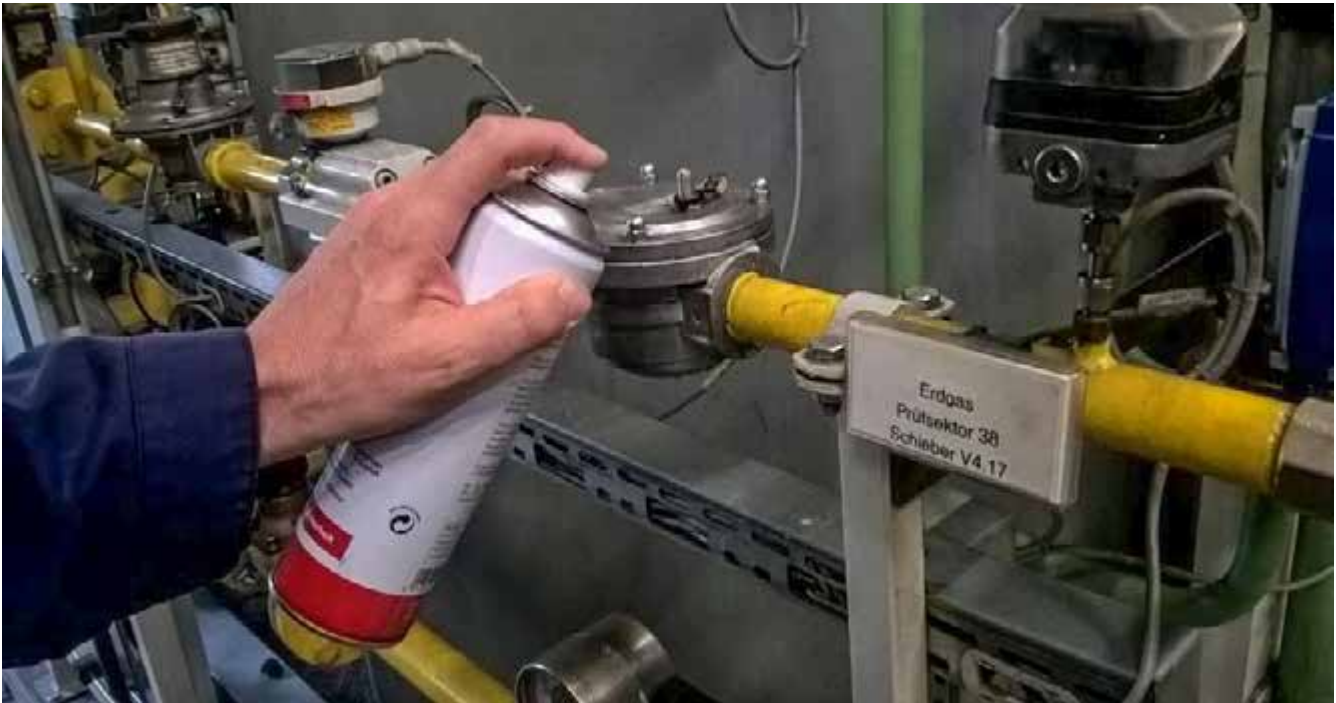
Figure 16 Leak detection by means of a leak detection spray
