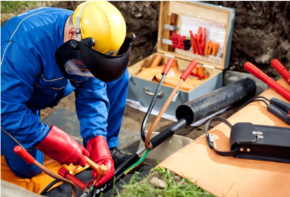
Fig. A 6-5 Installing cable sleeves: k_T = 1.9
