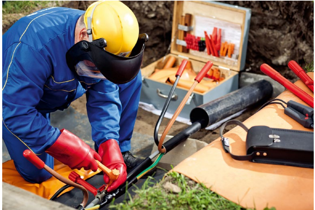
Fig. A 5-6 Working on a cable sleeve
