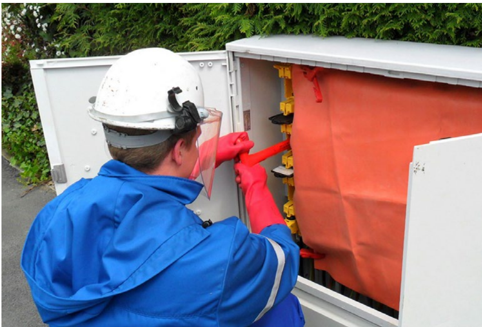
Fig. A 6-2 Replacement of a fuse panel in a control cabinet (close to the side wall): k_T = 1.0
