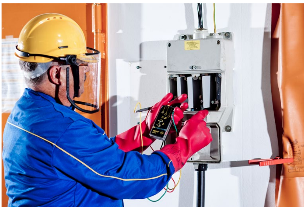
Fig. A 5-8 Working on a house junction box
