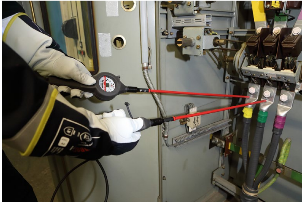
Fig. A 5-22 Determining a voltage-free state
