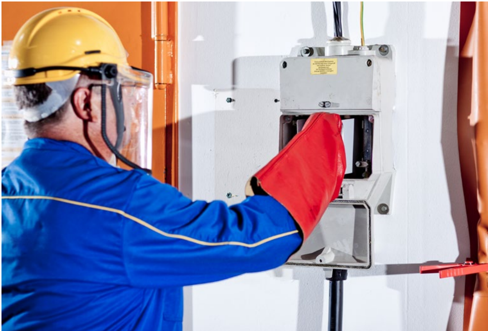
Fig. A 6-1 Working on a house junction box: k_T = 1.0
