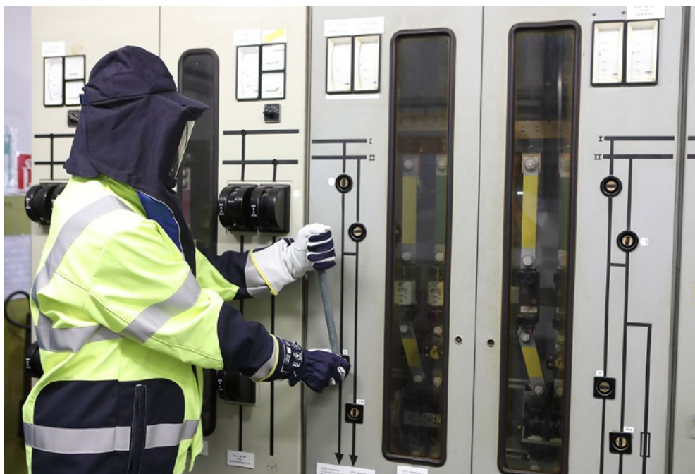
Fig. A 5-19 Opening the load break switch with a closed door by means of an operating lever
