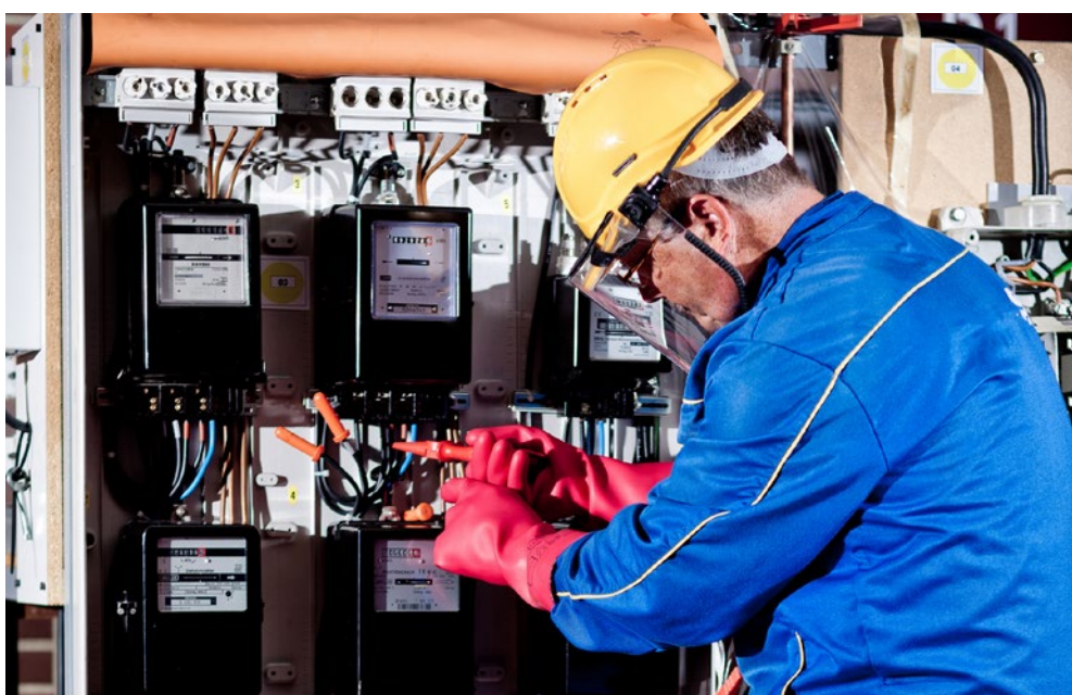
Fig. A 5-10 Working behind the house supply system
