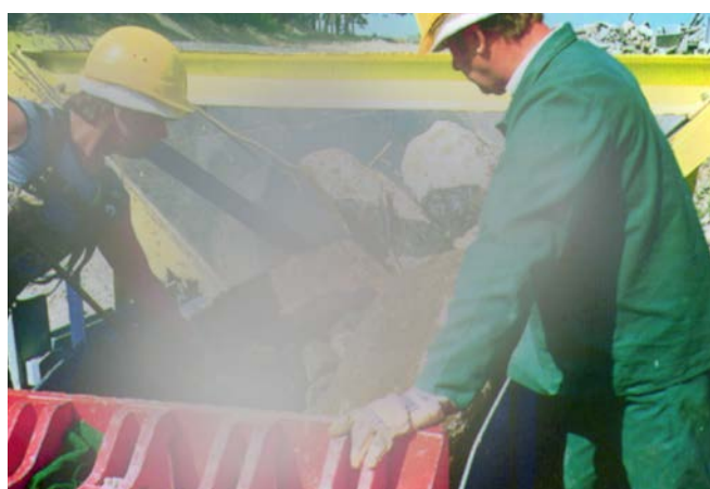
Figure 51: Manual removal of unwanted materials during recycling of construction materials
