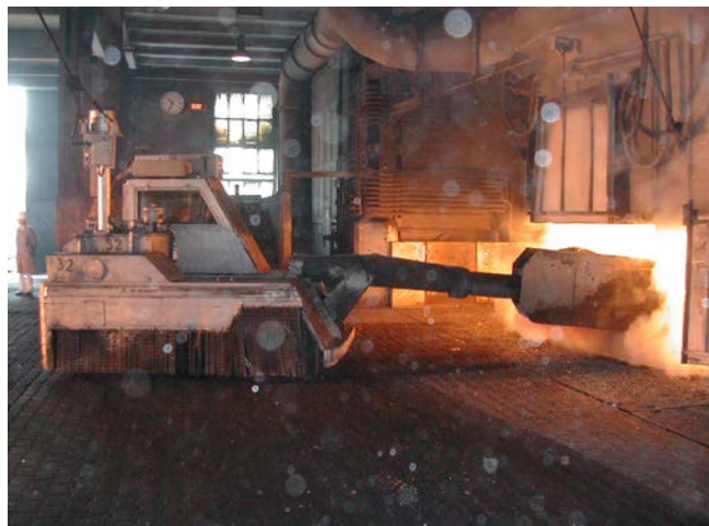
Figure 34: Electric furnace for the production of silicon compounds
