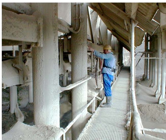
Figure 4: Inspection round in the ballast transfer area
