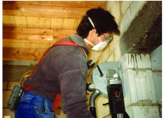
Figure 39: Cutting of chases for electrical wiring
