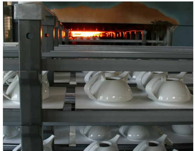
Figure 20: Tunnel kiln exit after firing. Source: VBG
