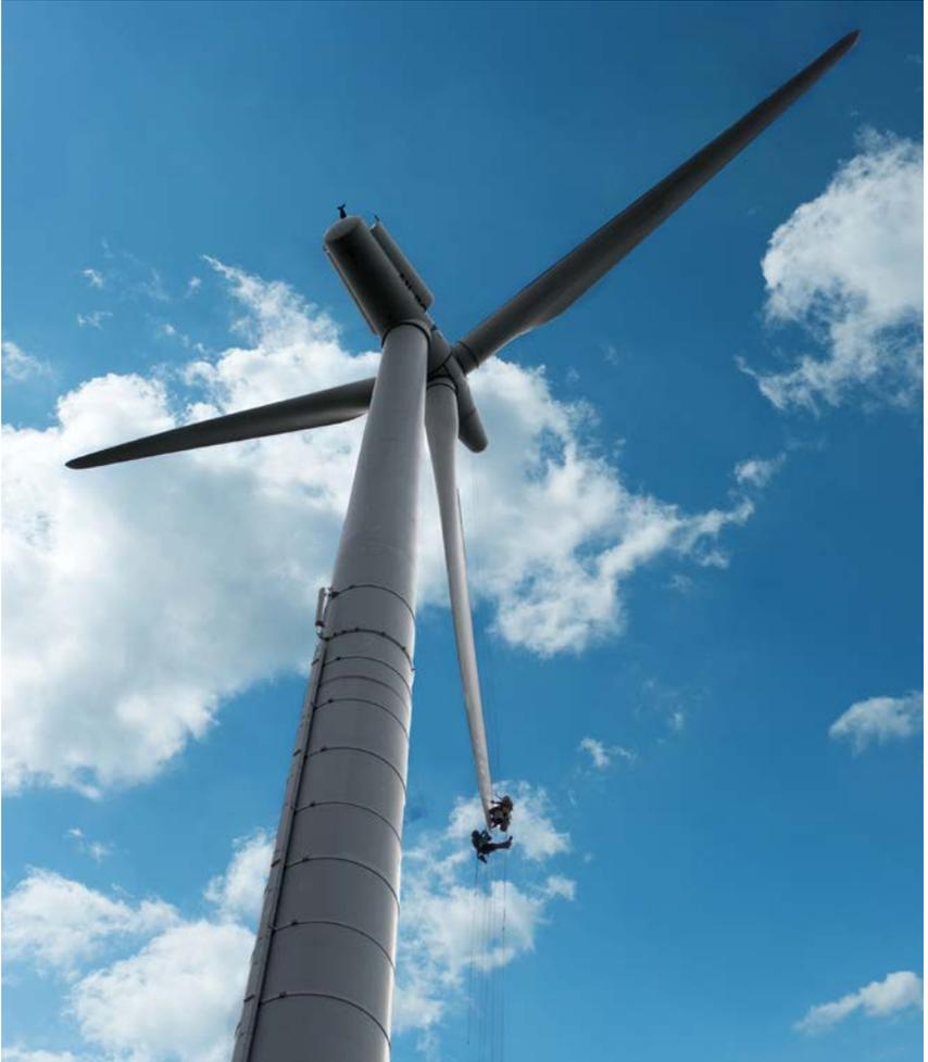
Abb. 43 Reparaturteam am Rotorblatt
