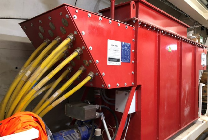
Abb. 10 Trafostation
