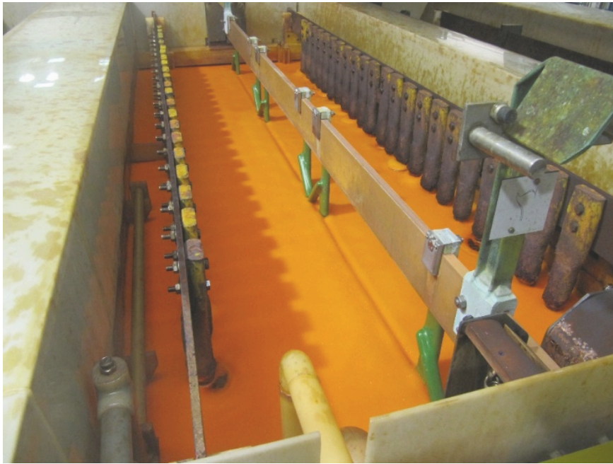
Fig. 10 – Chromium plating process tank with wetting agent on the electrolyte surface.
