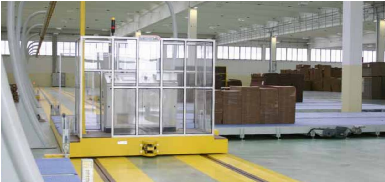
Visual or acoustic signals indicate the approach of a transfer car
