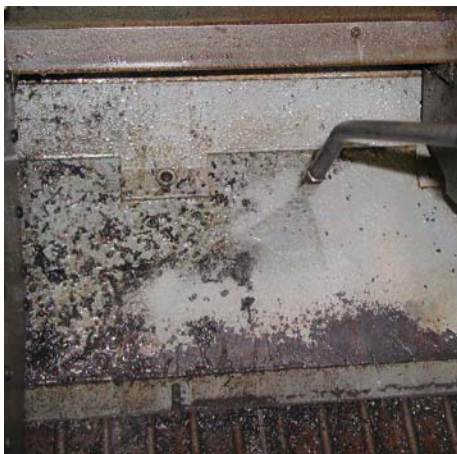
Figure 35 Cleaning with a low pressure device
