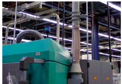
Figure 37 Connecting piece for vibration isolation: vertical, earthed
